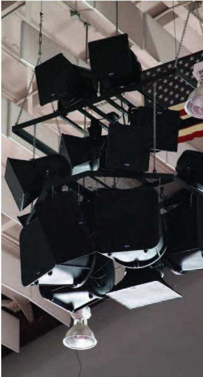
AH Horn clusters Can Provide Wide Coverage And High Output In A Variety Of Installation Types.
